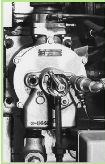
1813 Sensitrol Valve on a Dual-Fuel™ burner. Valve is used for setting ratio when burner is on oil; it is shut off when burning gas.
